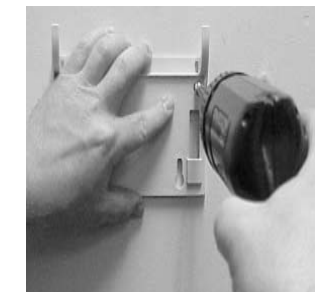
3. Drill holes for four wall anchors with a 5/16" drill bit. Use the mounting bracket as a template for proper spacing of the mounting screws. Install anchors, and then screw into anchors.
